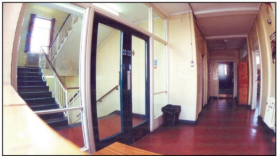
The Main Building (West End), 1 st Floor Landing outside Classroom 6.
